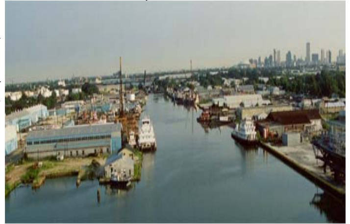
The Harvey Canal is an important location for many of the region’s oil field services.
