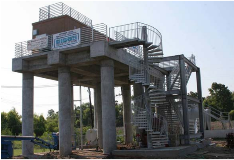
Safe House at Bayou Segnette Pumping Station
