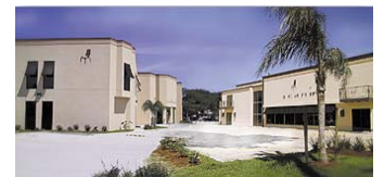
Scandinavia Furniture took advantage of the Restoration Tax Abatement program for the expansion of their building on Airline Drive.
