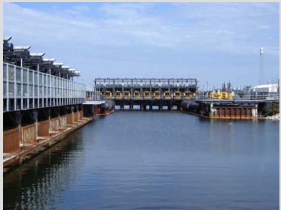
Major improvements to the hurricane protection system have been implemented since 2005.
