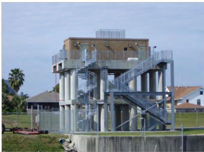
Major improvements have been completed or are underway to make Jefferson's pump stations, levees, and drainage system more resilient. Shown here is a new "safe house" for drainage pump operators.
