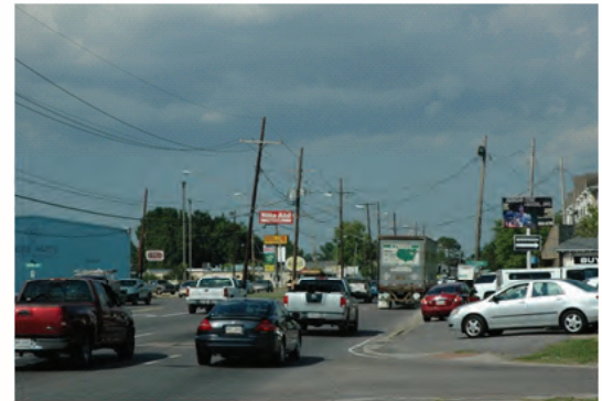
A maturing community with aging infrastructure, Jefferson has myriad transportation needs.
