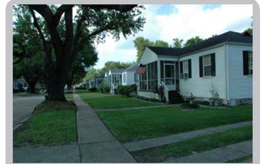
Impeccably maintained, tree-lined streets can be found throughout the residential neighborhoods of Jefferson
