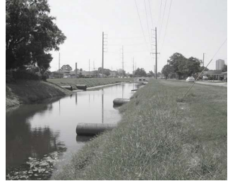
Existing condition along the canal
