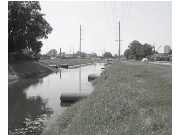
Existing condition along the canal
