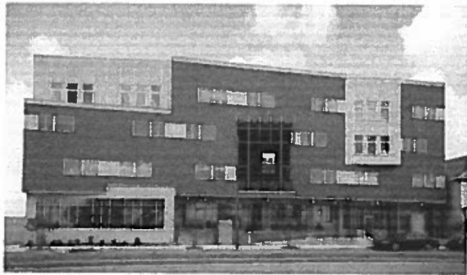
Photo 1. The Rosa F. Keller Building on Tulane Avenue
