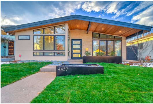
f. Covered entryway and roof overhang
