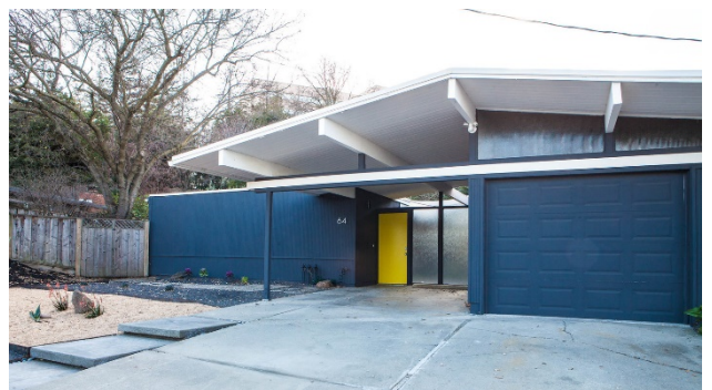
c. Exposed wood beams highlight the house's structural system
