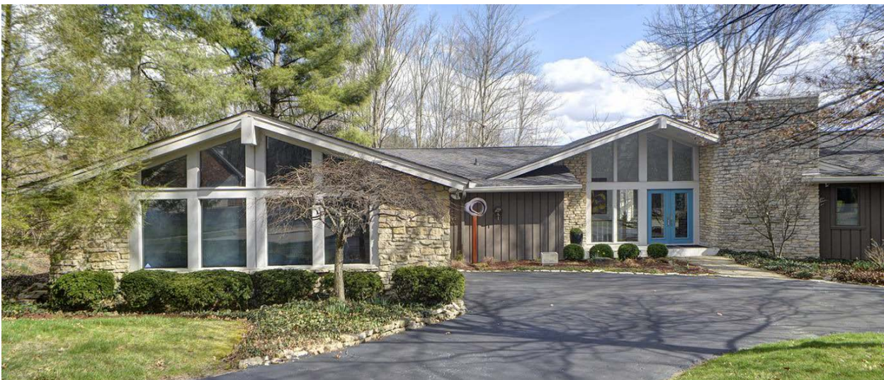
n. Curtainwall system used in floor to ceiling window and door design
