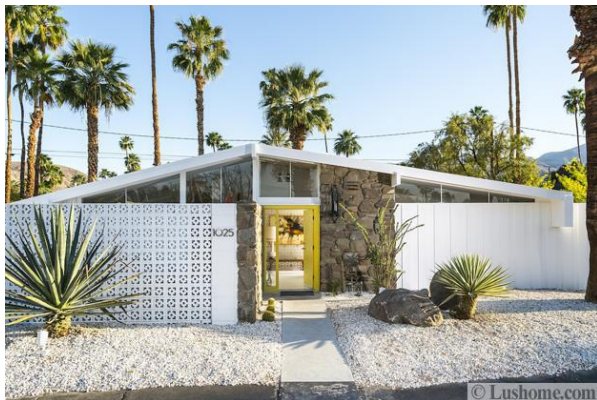
e. Solid entry door paired with clerestory and sidelight windows
