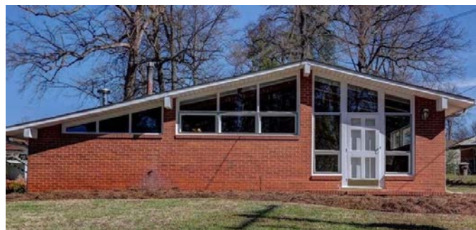
l. Single facade depth with little variation of materials
