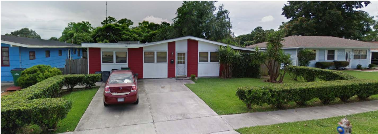
Typical Terrytown home with renovations
