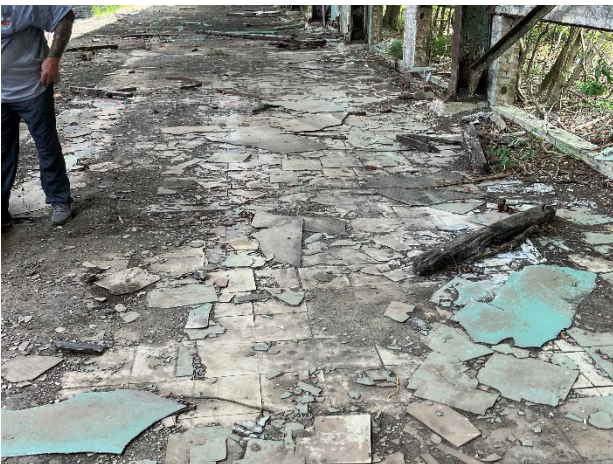
Photo of 12" x 12" Floor Tile and Mastic sampled in Factory Building.
