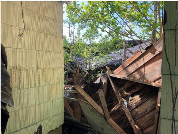
Photo of transite siding on the exterior of the Office Building.
