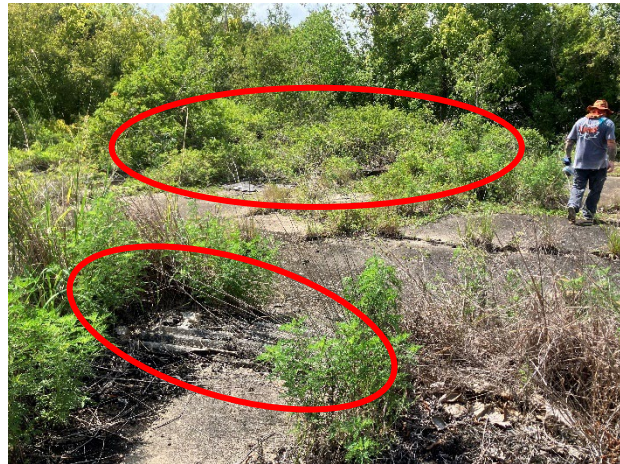
Photo of ACM building and construction debris.
