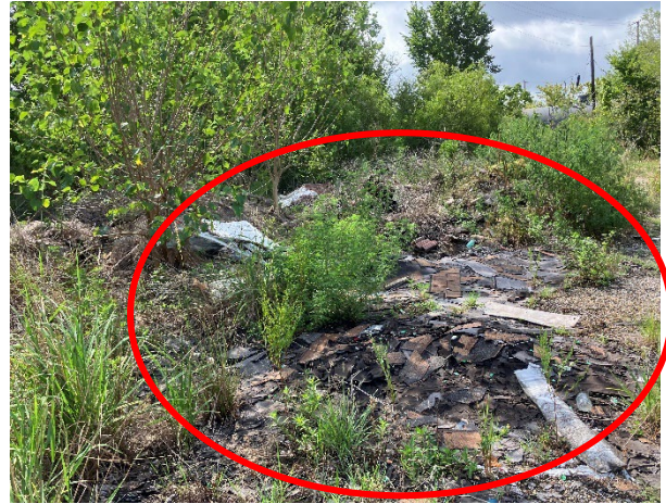
Photo of ACM building and construction debris.
