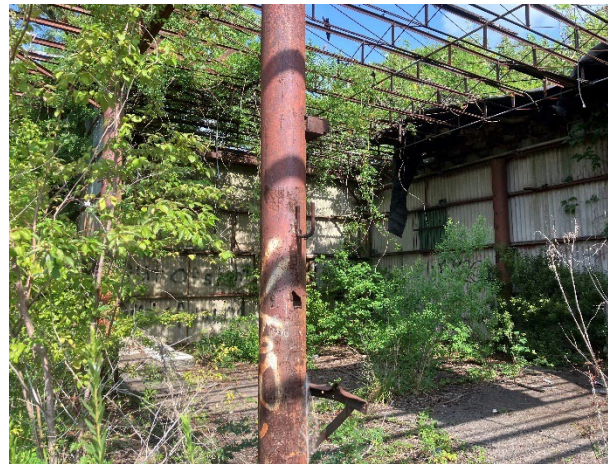
Photo of gray corrugated transite roofing and siding for the Cafeteria Building.
